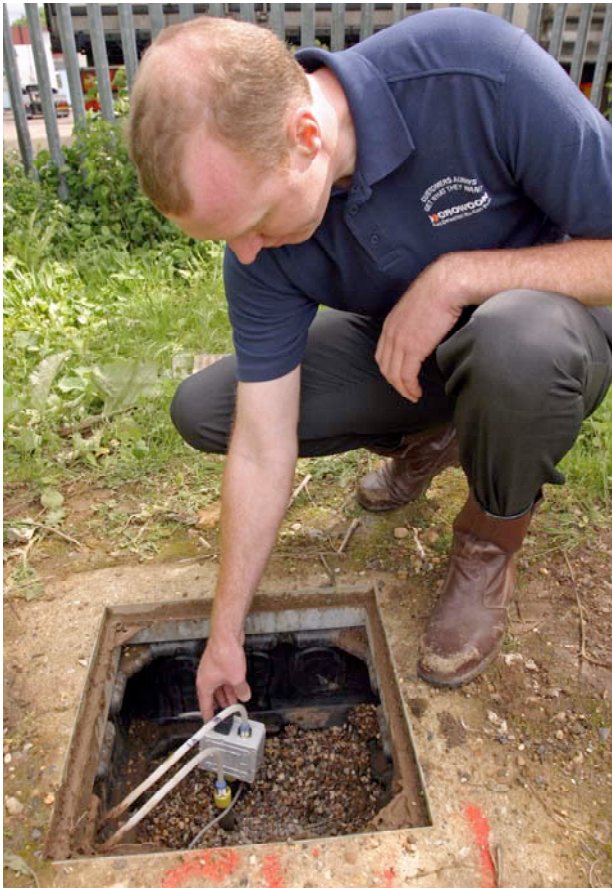
A borehole monitoring point with gas sampling tubes and a pressure transducer
