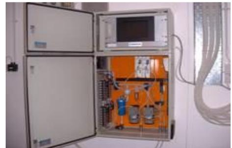
Two different types of gas sensor are used to monitor the biogas – infrared for methane and electrochemical for hydrogen sulphide. The methane measurement is in the range 0-100% by volume and is continuous.
