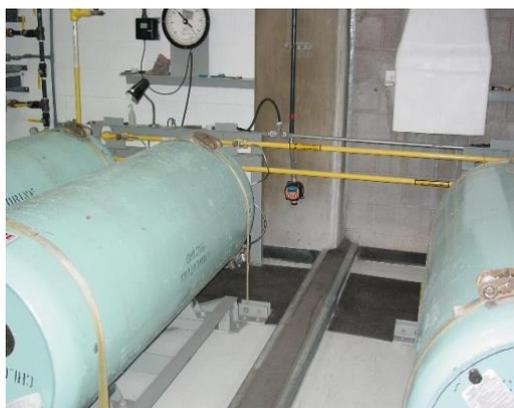
Storage areas for chemicals used within the final treatment stage should have robust gas detection systems installed; even small escapes of  $\text{Cl}_2$ ,  $\text{NH}_3$ ,  $\text{SO}_2$  or  $\text{O}_3$  can be extremely harmful.
